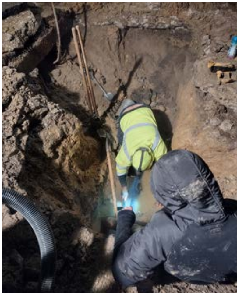
Small town, big problems as Winslow Water operators work to fix a water main break.
